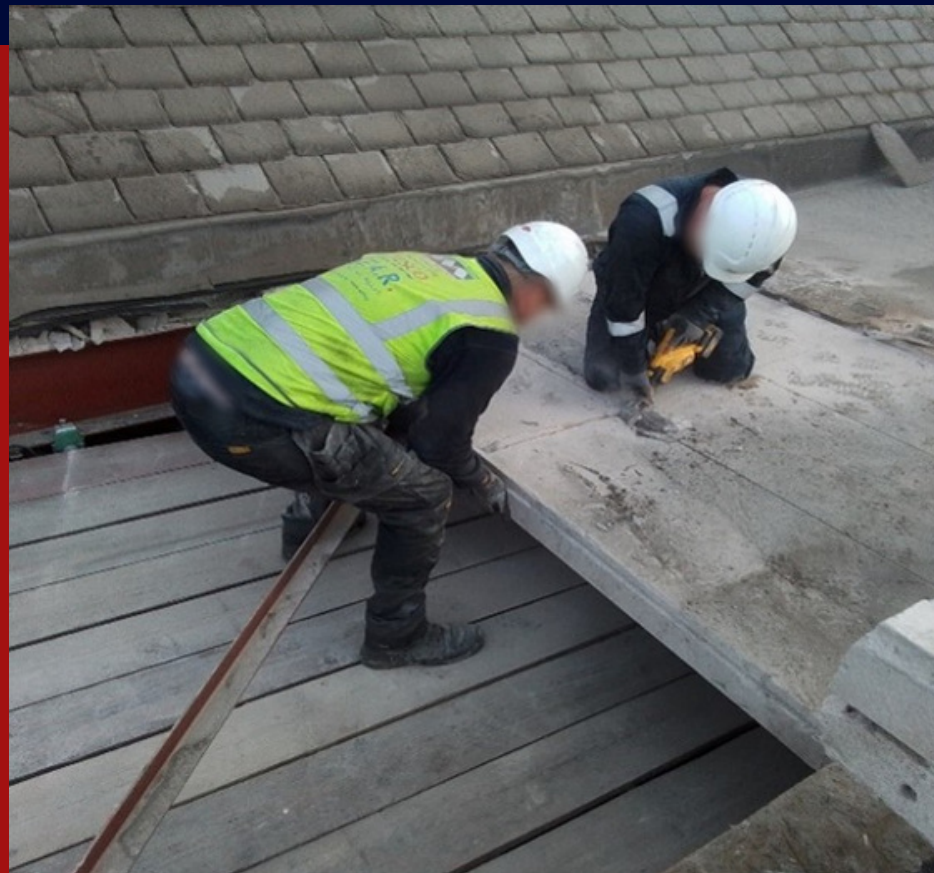
REMOVAL OF EXISTING RAAC PANELS
