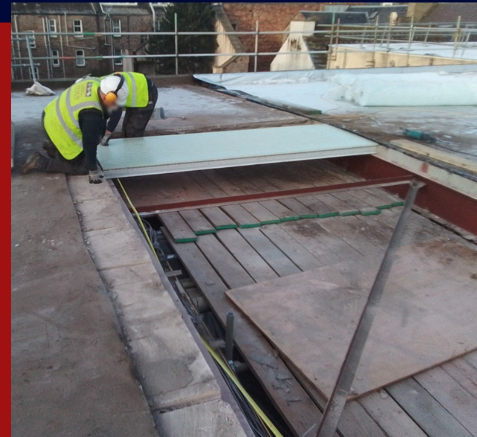
INSTALLATION OF NEW COMPOSITE DECKING PANEL
