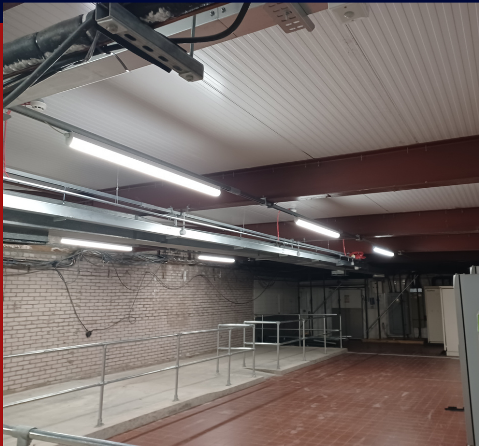
INTERNAL VIEW OF NEW DECKING PANELS
