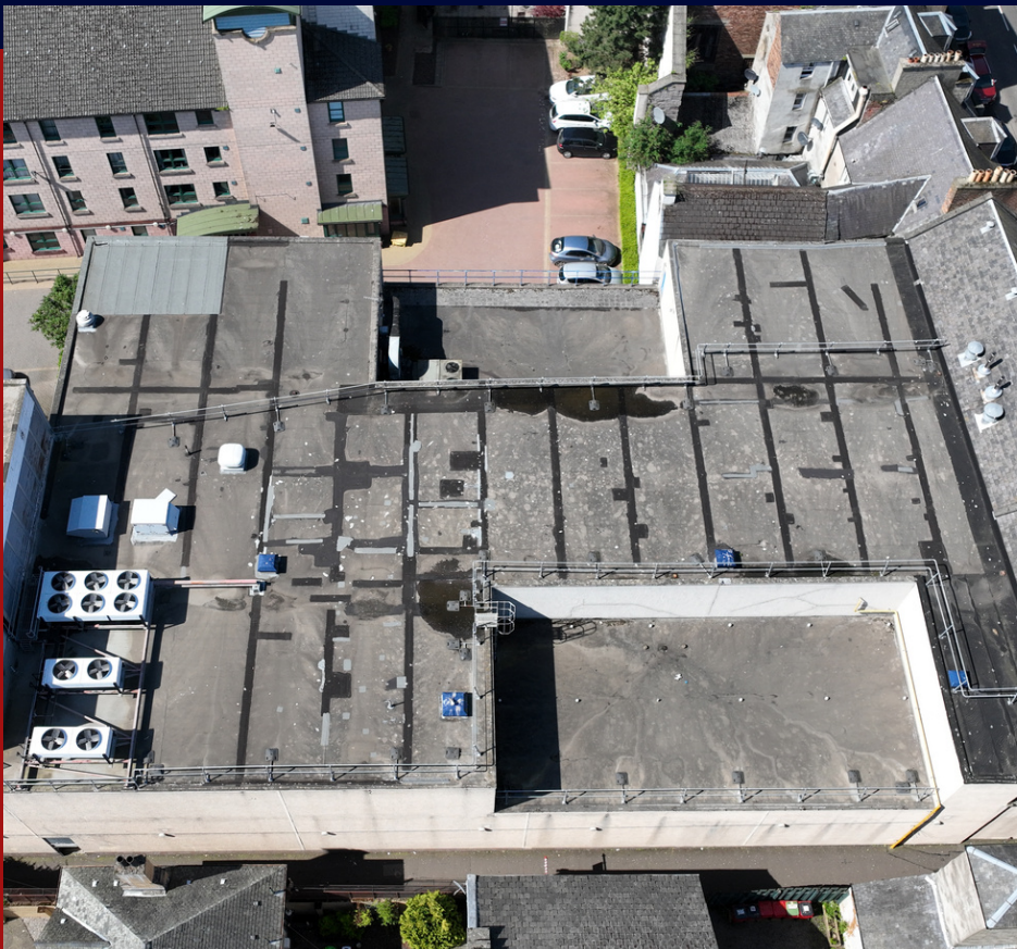
OVERVIEW OF EXISTING ROOF
