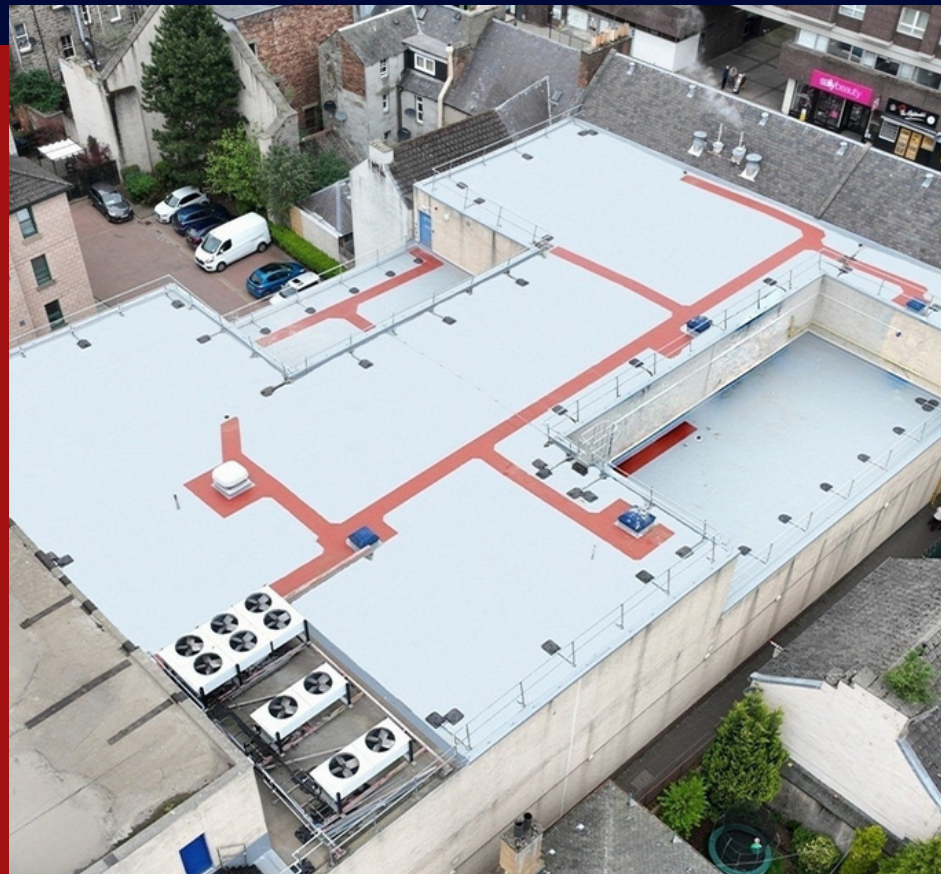
OVERVIEW OF COMPLETED WORKS
