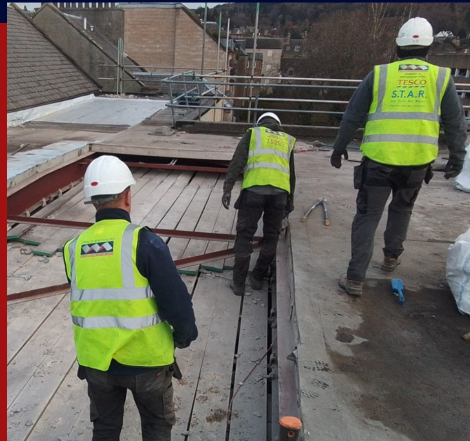
PREPARATION FOR COMPOSITE DECK INSTALLATION
