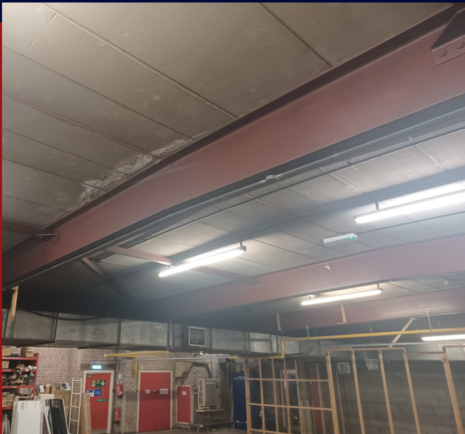
INTERNAL VIEW OF DAMAGED RAAC PANELS WITHIN WAREHOUSE AREA
