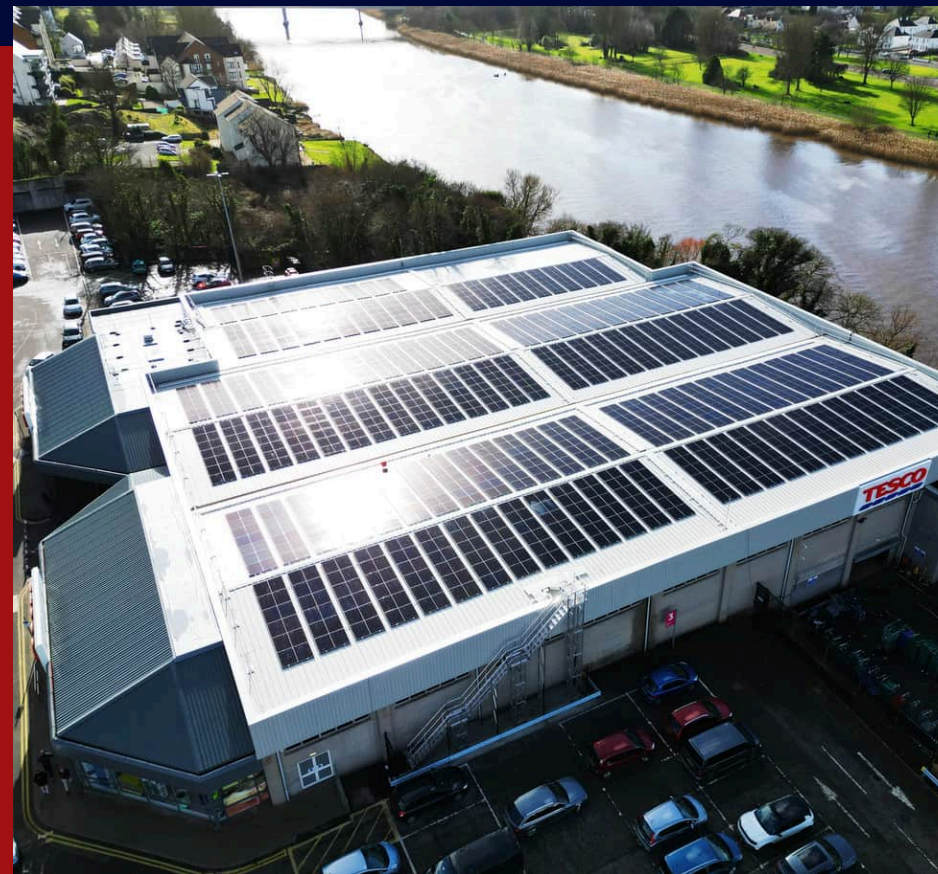
OVERVIEW SHOWING THE NEW ROOF AND PV SYSTEM
