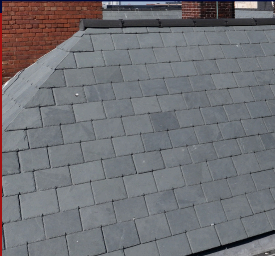
PORTION OF ROOF SLATES REPLACED
