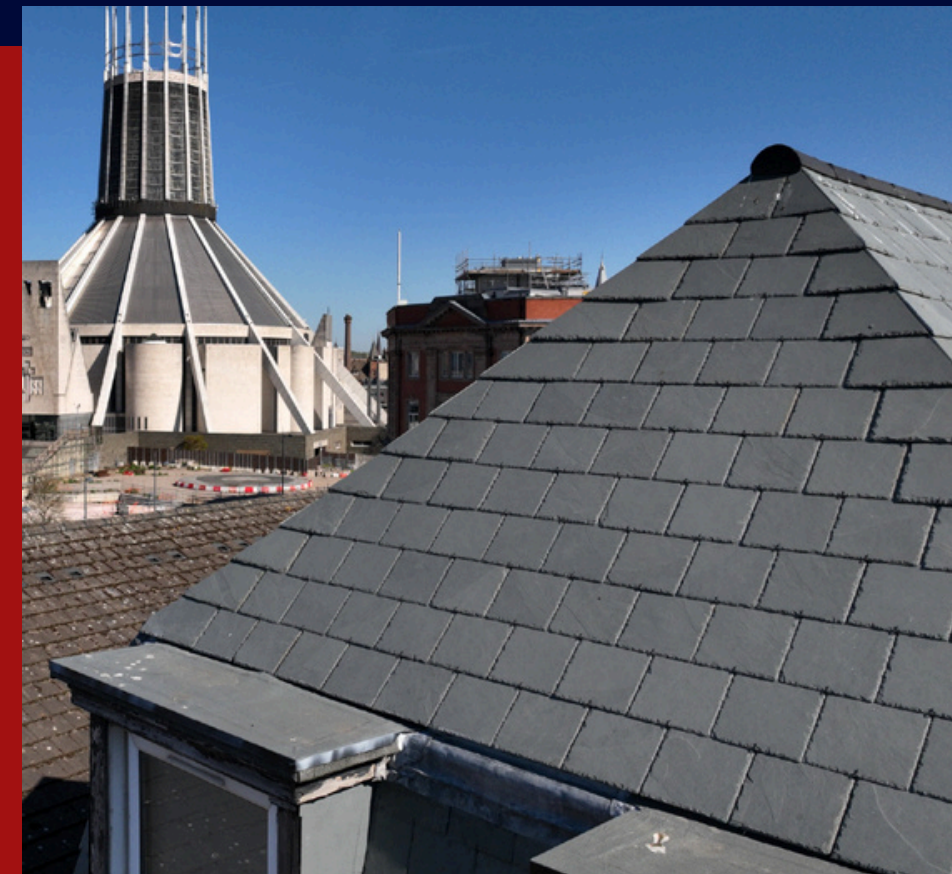
REPLACED ROOF SLATES
