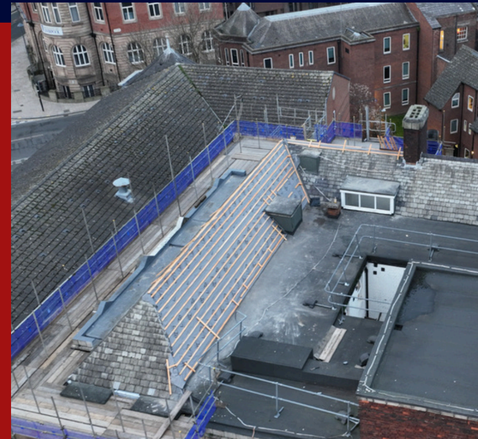
INSTALLATION OF ROOF BATTENS
