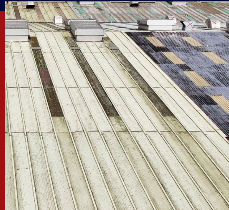
OLD COMPOSITE ROOF WITH FAIRS ROOF LIGHTS.
