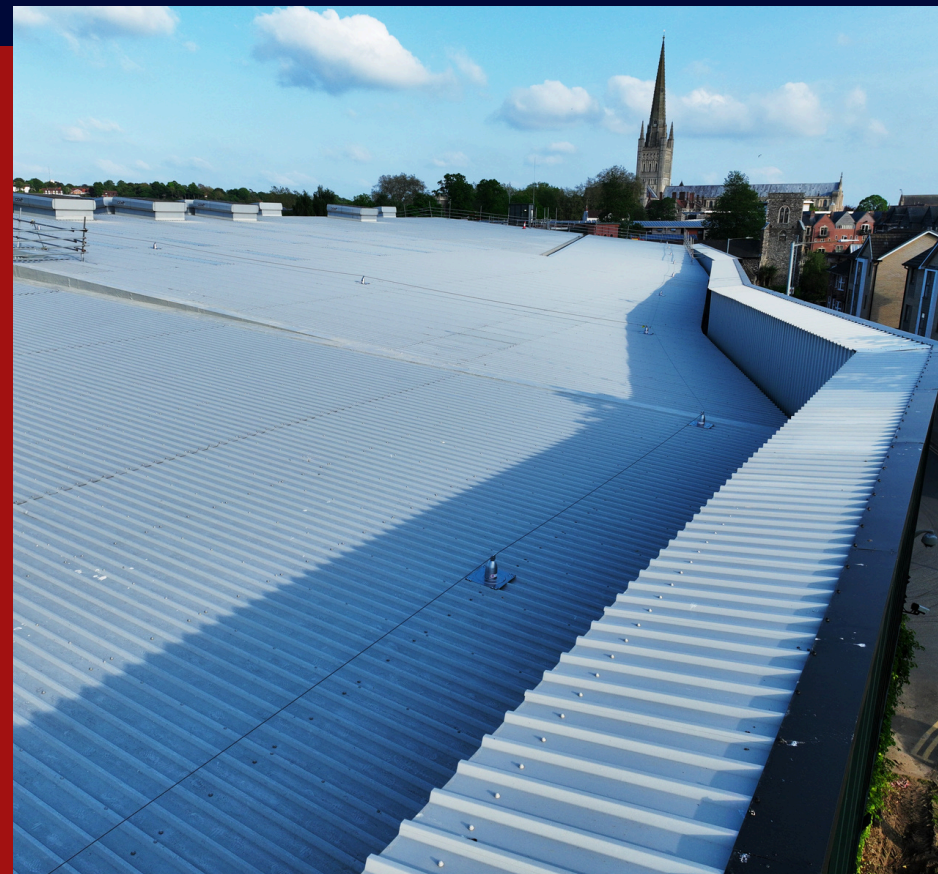
NEW BUILT U ROOF SYSTEM WITH CLADDED PARAPET WALLS.
