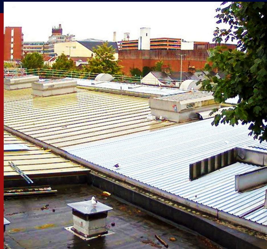
REPLACEMENT OF THE EXISTING COMPOSITE ROOF SHEETS.
