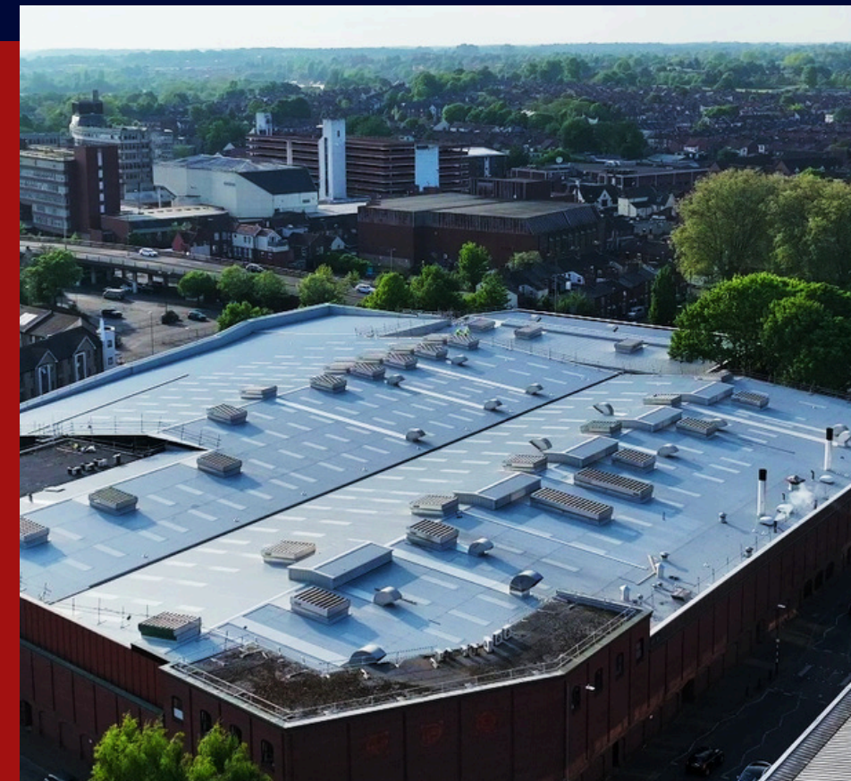
OVERALL COMPLETION OF THE PROJECT.
