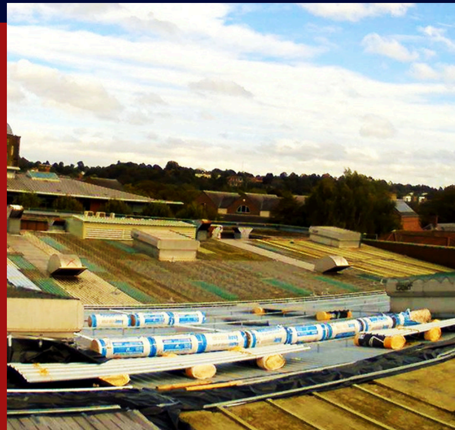
ONGOING REPLACEMENT OF THE EXISTING ROOF.
