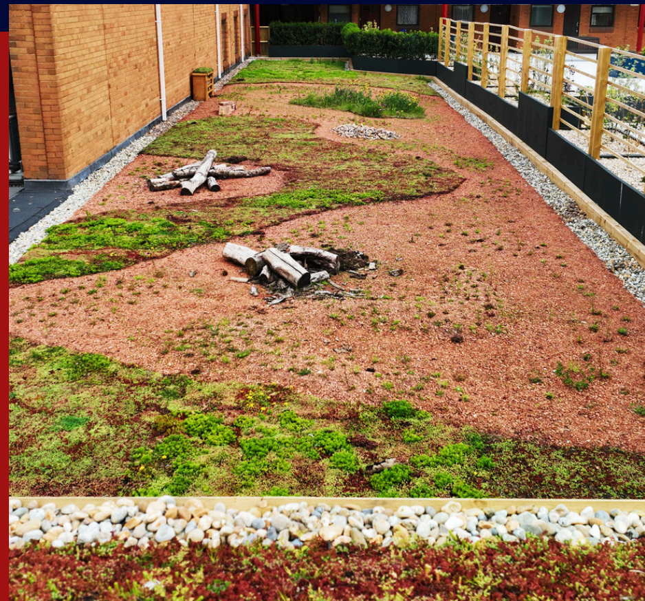
GREEN ROOF AREA OUTSIDE THE TESCO COLLEAGUE ROOM
