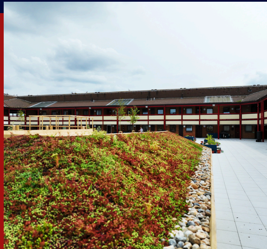
GREEN ROOF COVERING OF THE NEW BIN STORES
