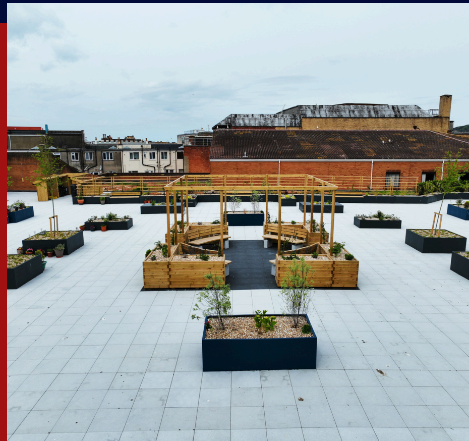
OVERVIEW OF THE ROOF AND PLANTERS
