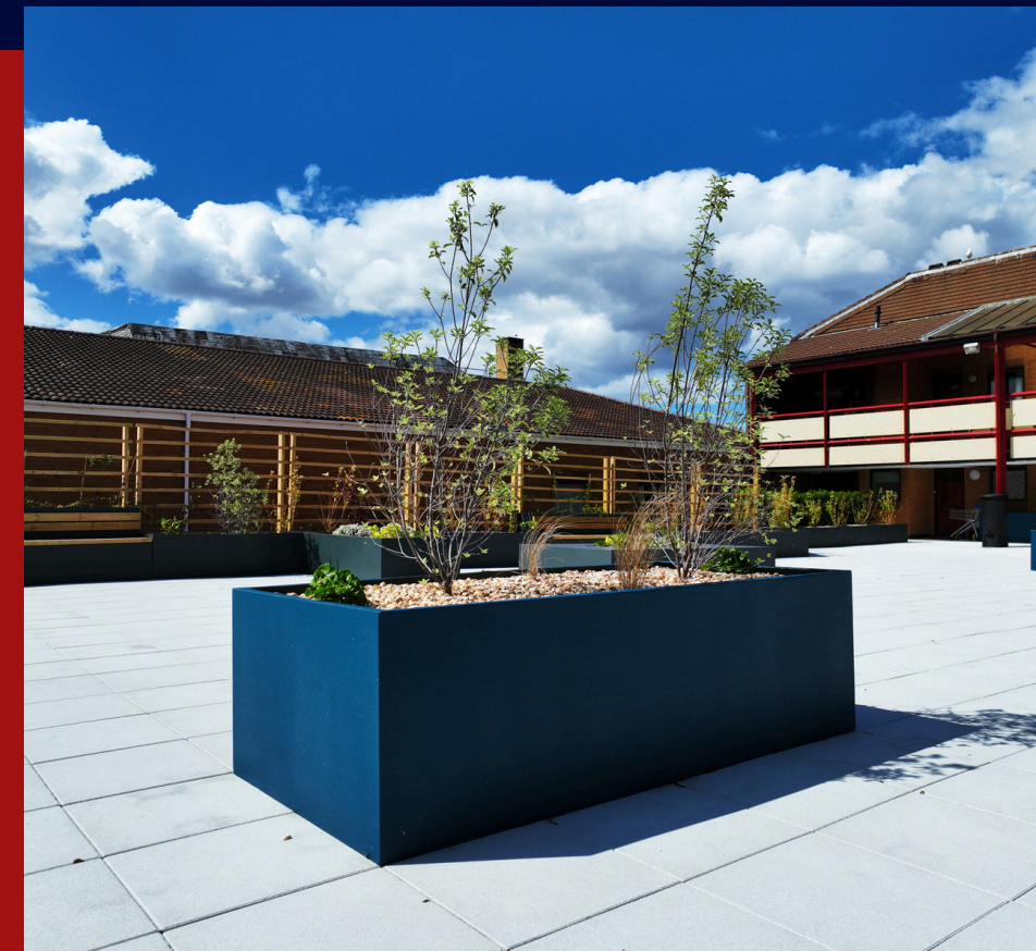
NEW PURPOSE-MADE, LIGHTWEIGHT PLANTERS WERE INSTALLED FOR RESIDENTS TO USE
