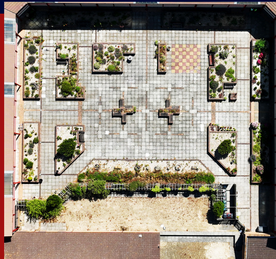
OVERHEAD HIGHLIGHTING EXTENT OF THE EXISTING SLABS, PLANTERS.
