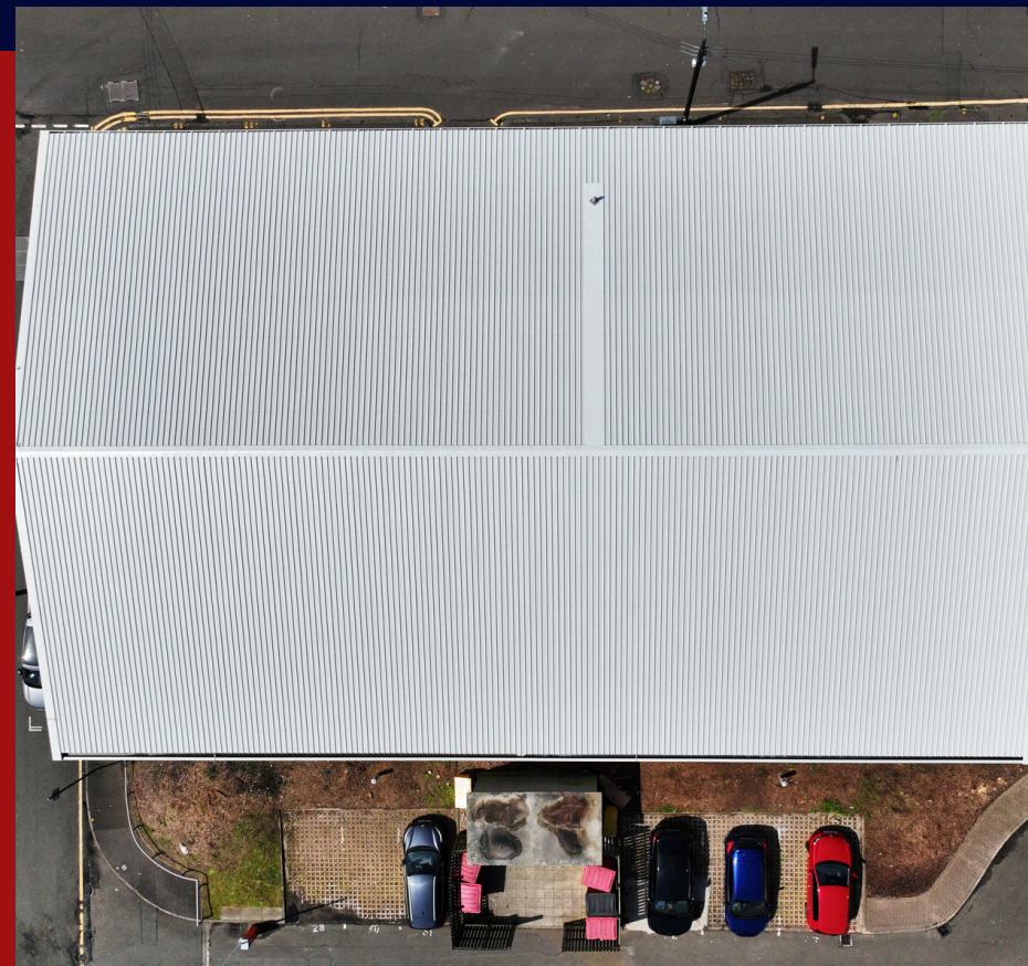
COMPLETED ROOF SYSTEM
