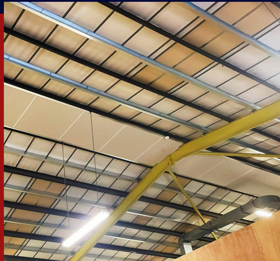
INSTALLATION OF INTERNAL STEELWORK
