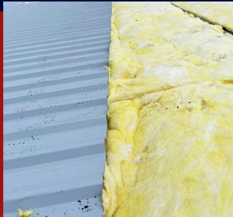
INSTALLATION OF INSULATION
