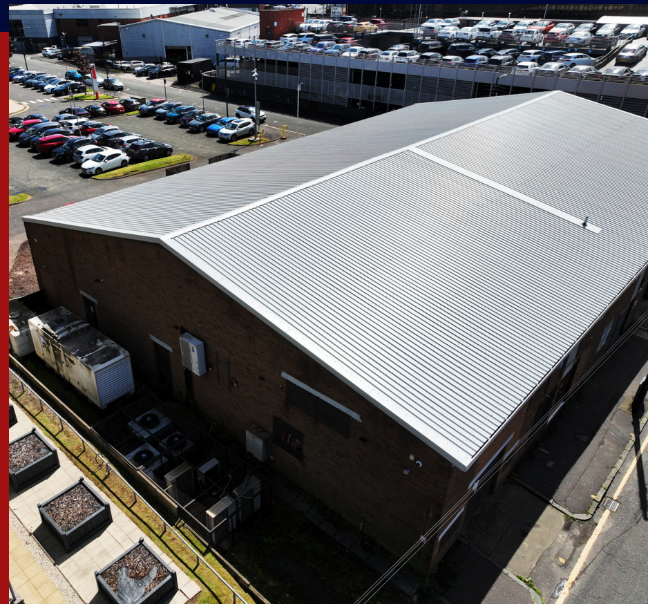
COMPLETED ROOF SYSTEM
