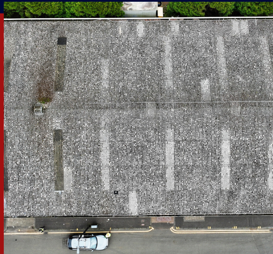
EXISTING ASBESTOS CEMENT ROOF
