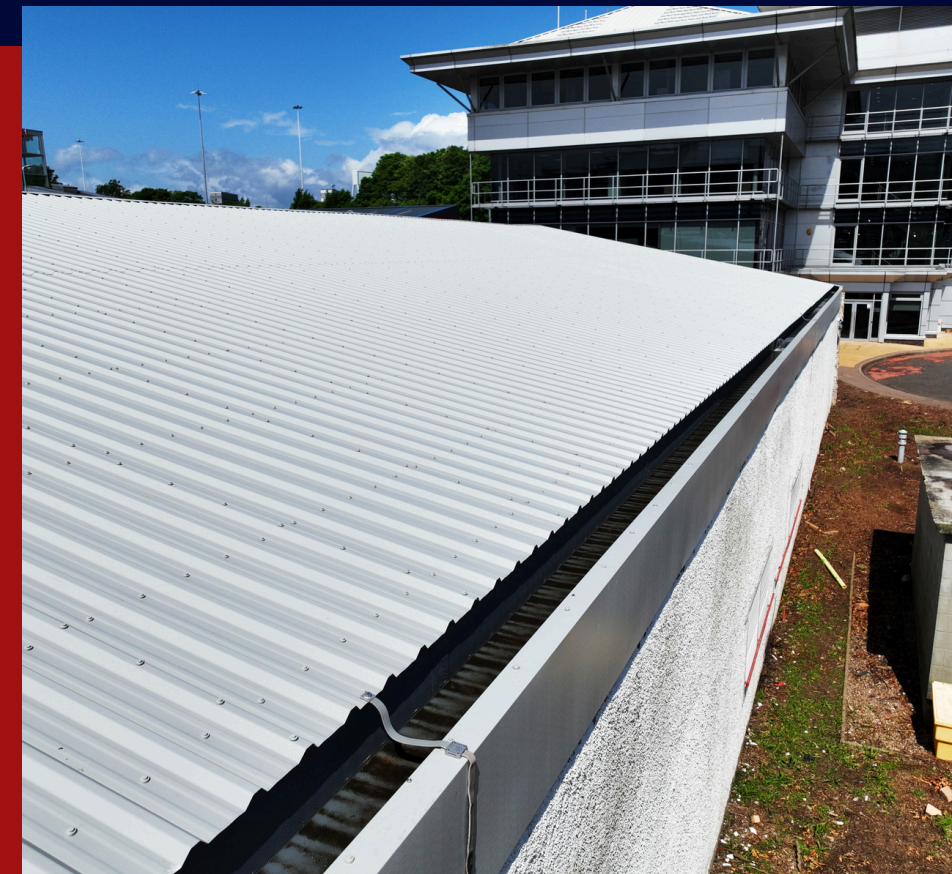
NEW GUTTER INSTALLATION
