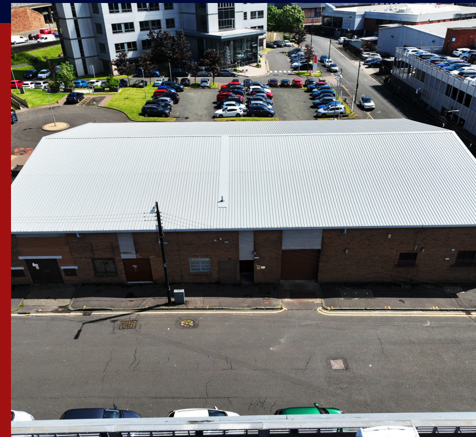
COMPLETED ROOF SYSTEM
