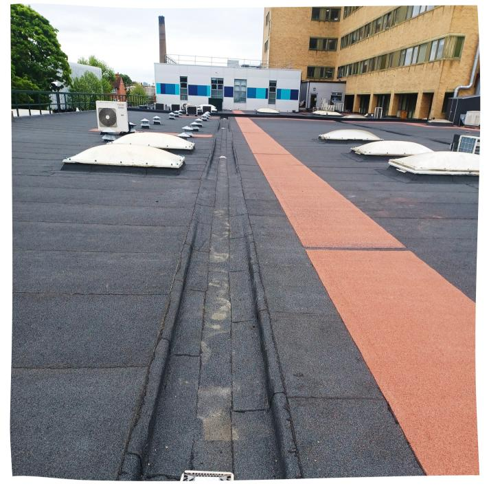
Overview of the roof following works, sumped gutter and clearly demarcated walkway.
