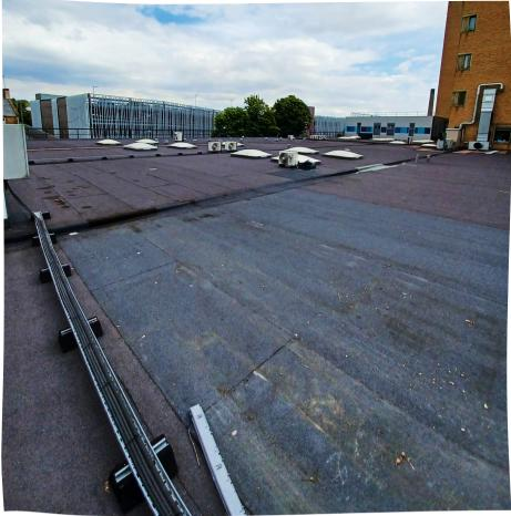
Before works, the image shows the condition of the felt, blisters, and failed laps.
