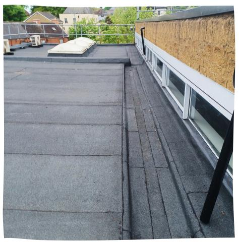
Sumped gutter detail around the edge of the building carefully designed and detailed.
